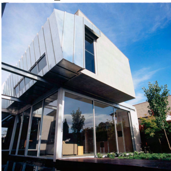
The street-facing "pod" (above) gives way to a light-filled entry and open-plan kitchen (above, left). Glass doors open onto a stylish barbecue area at the back (left).
