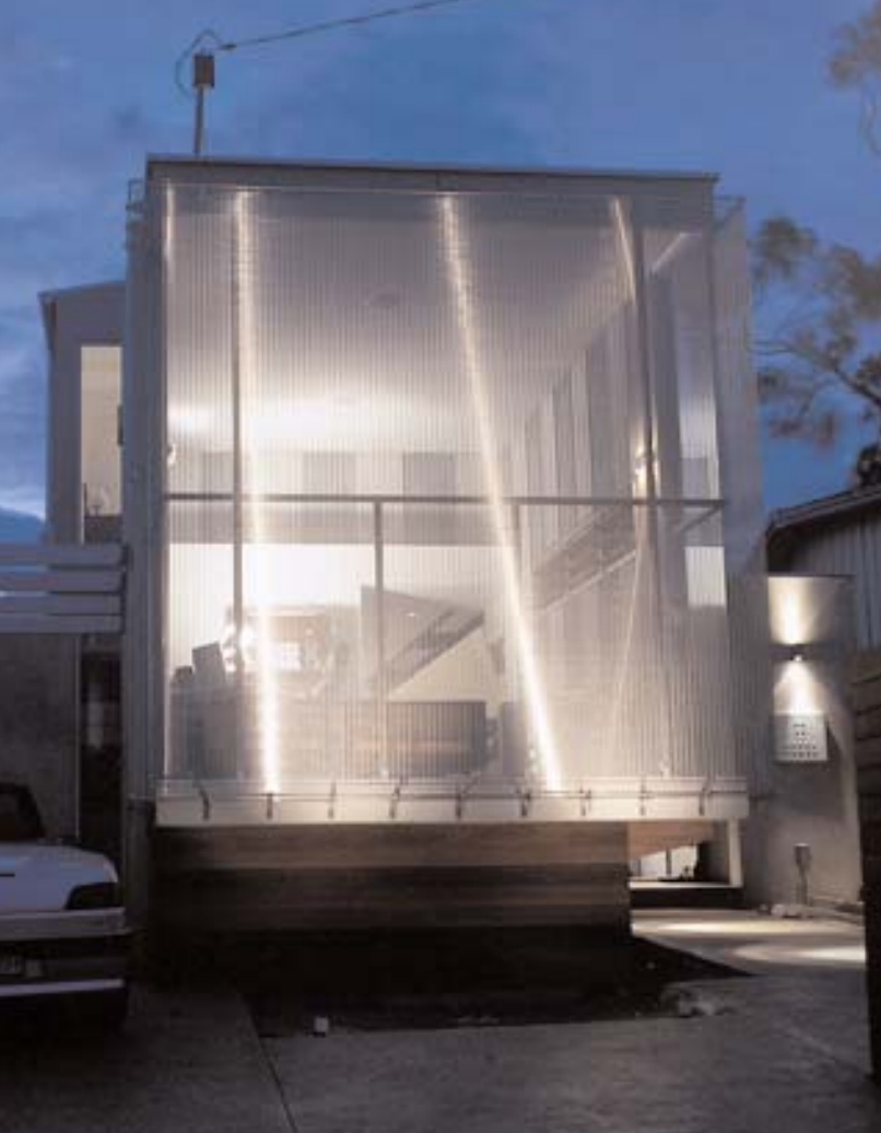
LEFT: When internal lighting is switched on after dark, the stainless steel mesh facade becomes translucent.
